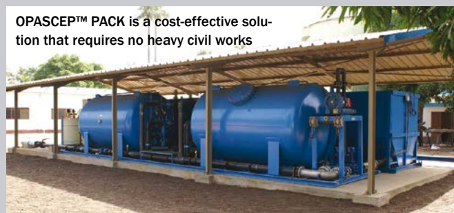
OPASCEP™ PACK comprises skid-mounted systems that turn surface water into drinking water
