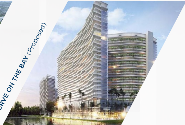
Residential 112-130 NE 41 Street
