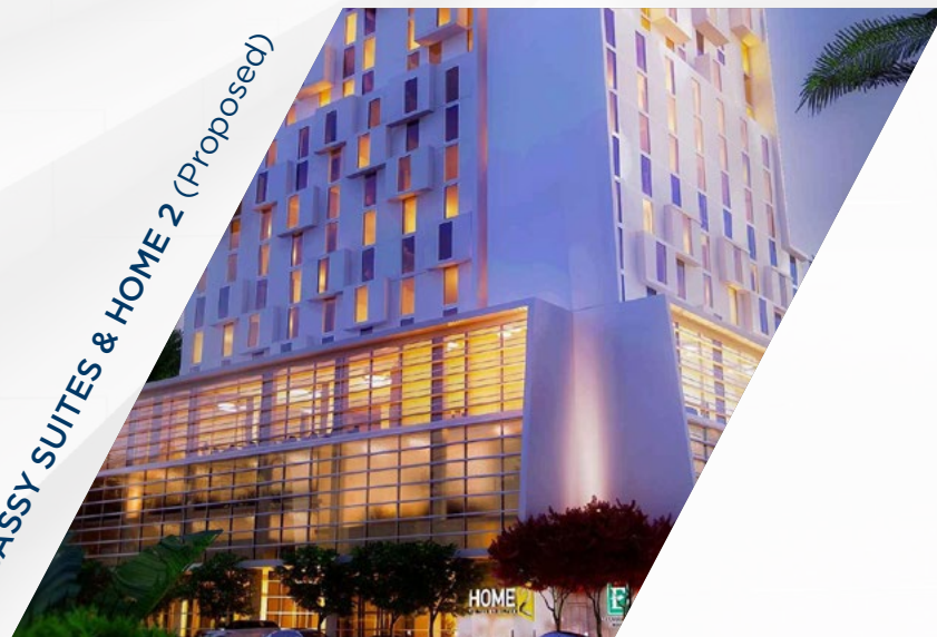
Hotels (Hilton brands) 1129 SW 3rd Ave.
