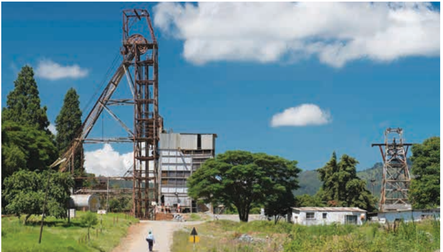
Redwing, one of Zimbabwe's historic gold mines. It has been flooded in recent years but dewatering has now been completed and it will re-enter operation later this year (photo: Metallon).
