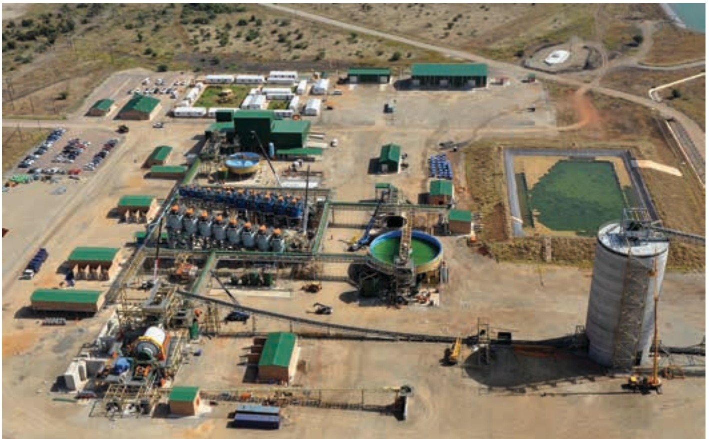
Recent photo of the Maseve processing plant. It has a capacity of 110 ktpm but allowance has been made for this to be increased to 160 ktpm (photo: Platinum Group Metals).
