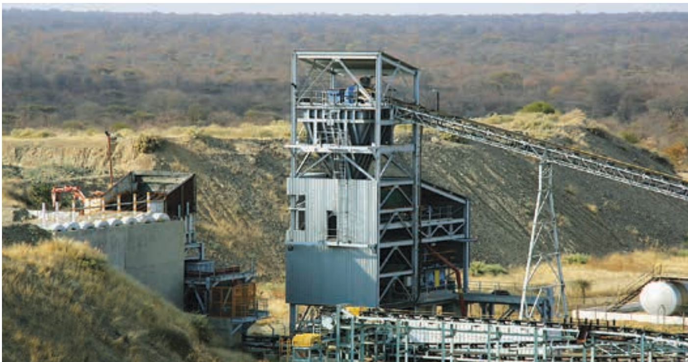
The Lerala mine showing the crusher installation (photo: Kimberley Diamonds).
