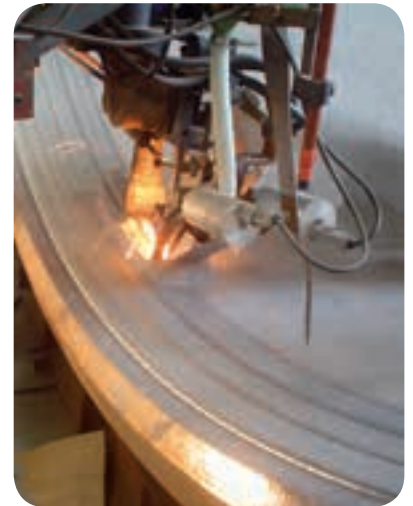
Electro-slag welding (ESW) single layer cladding using UTP Soudotape 825 in combination with Record EST 138 flux. The ESW process enables the required surface chemistry to be achieved in a single layer on certain applications.
