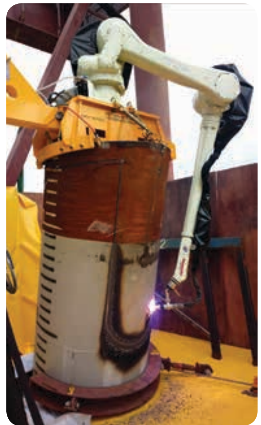
Figure 3: The robot system plasma cutting and bevelling a pile.
