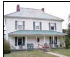
MLS 44431 - Elk Creek - 5 BR, 1 BA, HW floors, fireplace, metal roof, outbuildings. $74,550 (4 additional ac. available for purchase)
