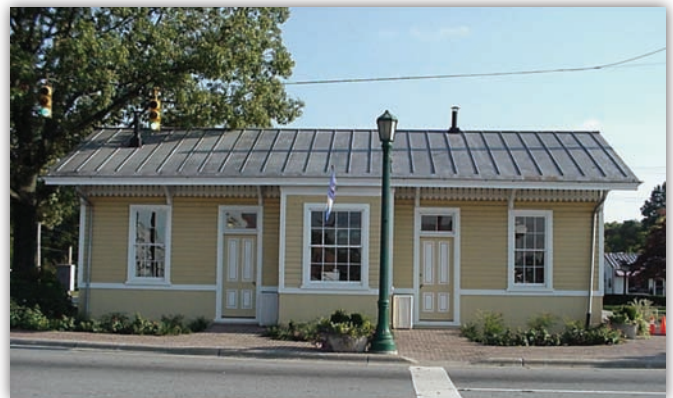
The Town Center Plan identifies a possible site for a reconstructed train depot like this one that exists today along the North Carolina Railroad in Thomasville. (Photo courtesy of the City of Thomasville)
