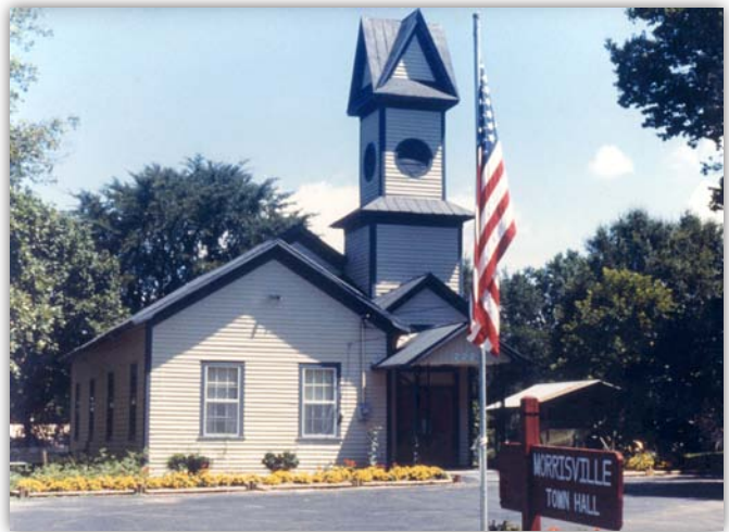
To help catalyze the restoration of the historic crossroads village, the Town Center Plan calls for restoring the old Christian Church and making it available once again for use by the community. (Photo: Town of Morrisville )
