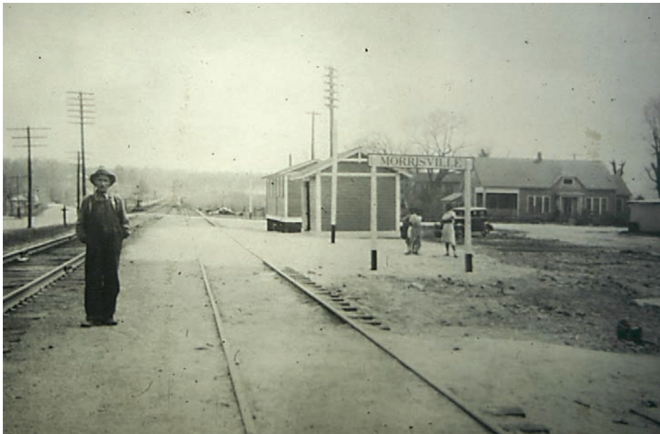
Image of depot taken in the 1930's looking south.
