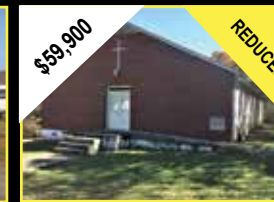
MLS# 54859 SPEEDWELL Brick church with over 3200 SF of space on 1.03 acres w/ an extra building on property.
