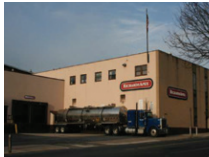
▲ The Richards Apex production plant
