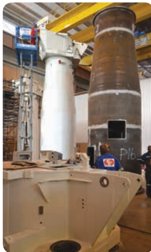
Efficient Engineering’s current flagship project is the fabrication and full electrical and mechanical integration of the yokes and pedestals for the first 64 Meerkat antennas for the Square Kilometre Array (SKA) project.
