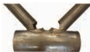
Figure 11: A tubular K-Joint after preparation for the hole drilling method.
