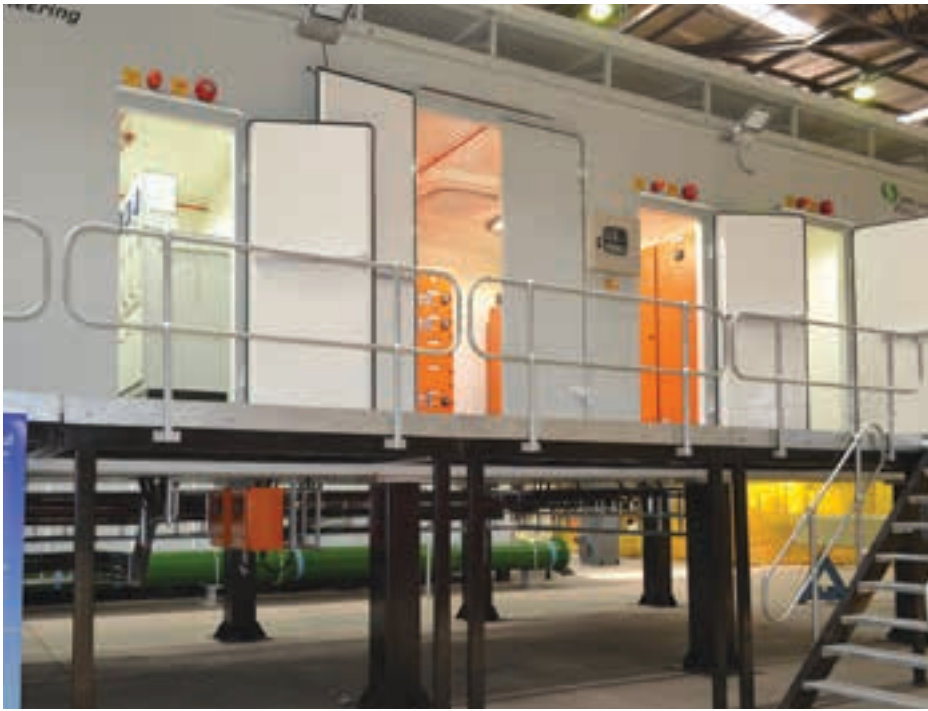
Above: The complete pump station, which was fully tested and commissioned on the factory floor of Efficient Engineering's Tunney premises, was delivered to the Sishen site and then deployed and anchored to the plinth in only three days.
