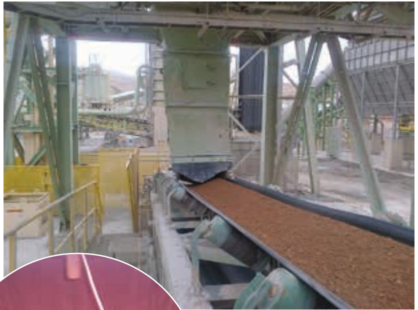
Above: Control of material from the transfer point will optimise belt life.
