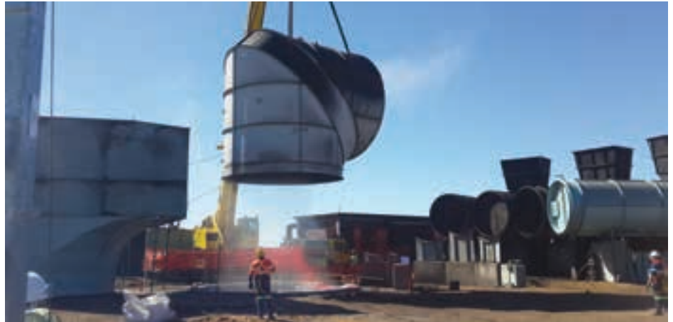
The new shaft top being lowered into place over the mouth of Black Rock mine's 500 m deep main ventilation shaft.
