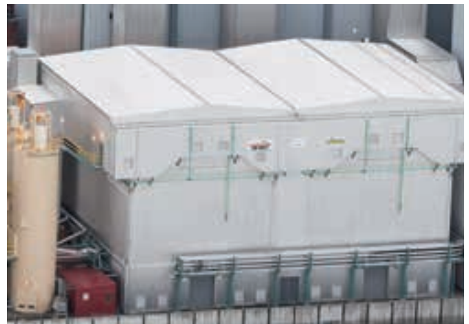
Clyde Bergemann's retrofitted pulse jet fabric filters feature: a patented stepped inlet manifold design for uniform gas distribution and reduce pressure drop; a patented inlet vane system to uniformly distribute gas flow and reduce bag wear; lower total pressure drop, which reduces I.D. fan power consumption and operational costs.
