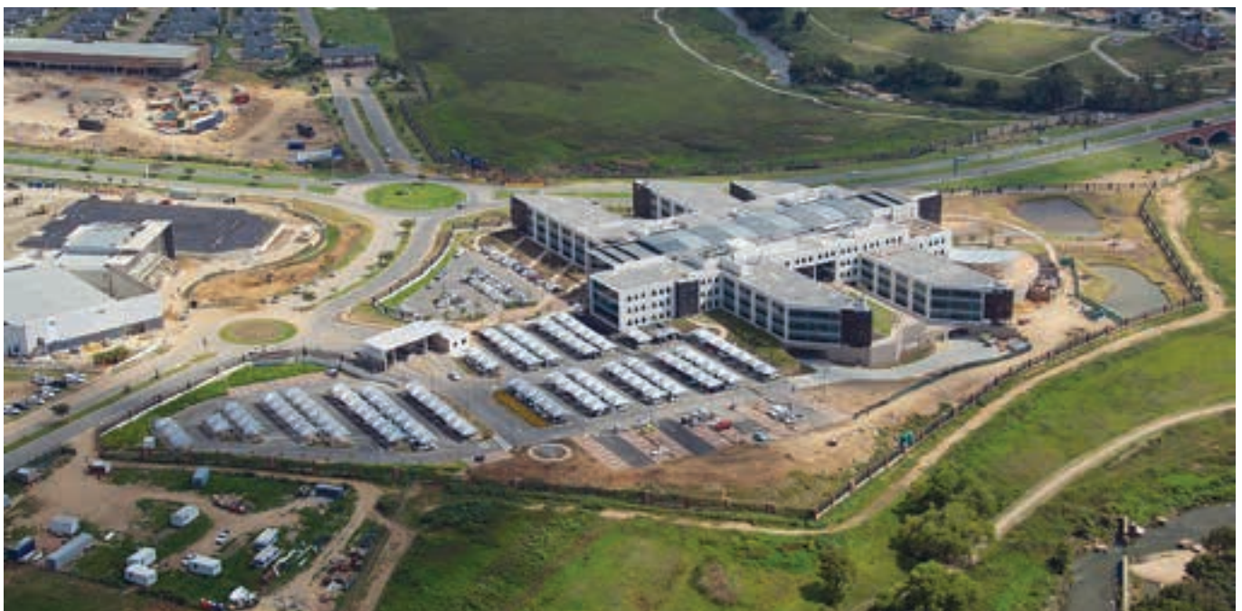
An aerial view of Group Five's 5 Star Green Star building on the Waterfall Estate in Midrand.
