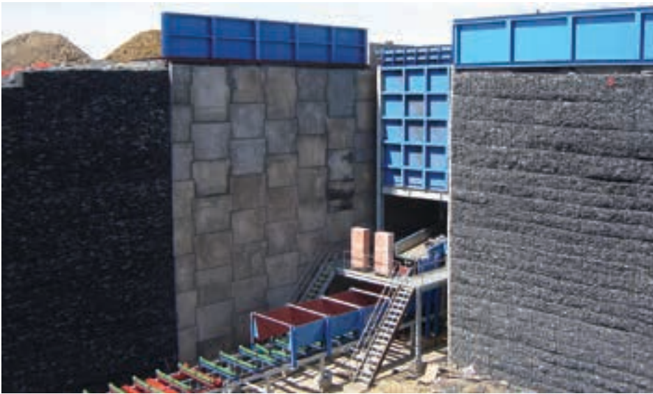
Above: MacRes and Terramesh tip wall at Optimum colliery.
