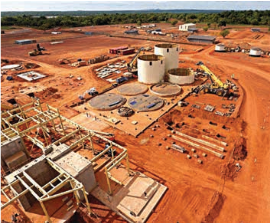
The process plant at Sissingué under construction (photo: Perseus Mining).
