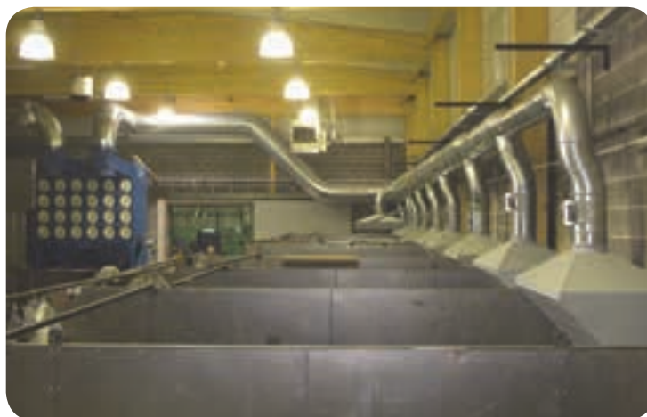
Donaldson's collector units can be combined in various configurations to make up larger units with air volumes ranging from 2 500 m 3 /hr to 200 000 m 3 /hr.
