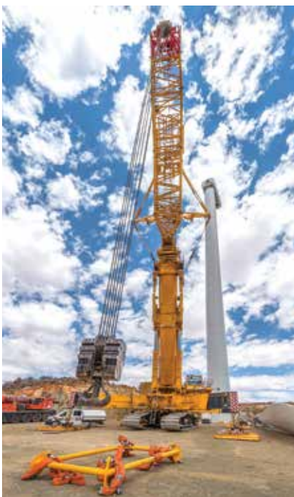
ABOVE: Johnson Crane Hire’s LTR 11200 crawler crane in action.
