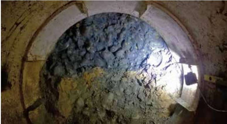
Treated jacking face holding cobbles and fines in suspension.
