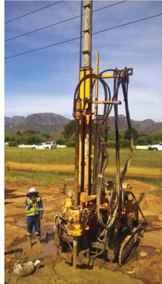
Jet grouting rig alongside N1.
