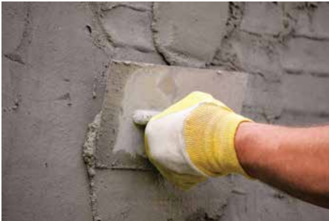
Chemical solutions company CHRYSO Southern Africa recommends the use of CHRYSO® Stab rather than water in order to retain workability of plaster or mortar.
