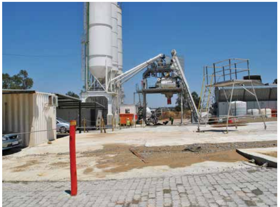
LEFT: Mohamed Docrat, production superintendent at AfriSam's Jukskei Quarry showing some of the paving work done using recycled concrete. RIGHT: The return concrete has also been used around the readymix plant to pave large areas.
