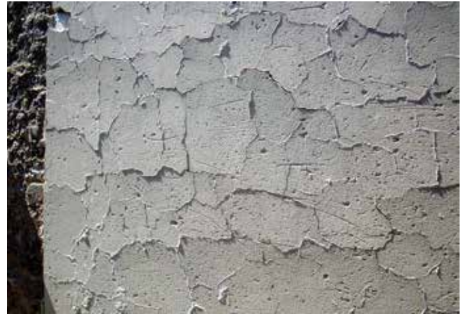
Plaster popping as a result of expansion of ash bricks.
