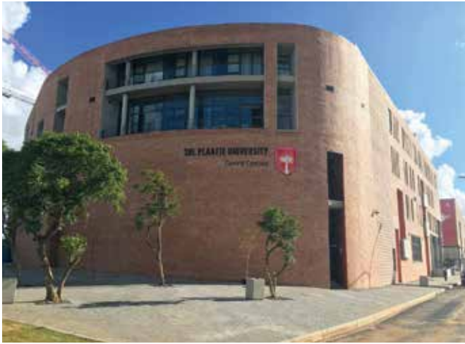
AECOM was appointed to provide project management services relating to the development of the Sol Plaatje University.
