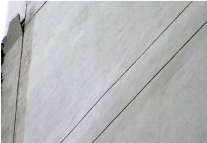
Debonding of plaster is often noticed as a hollow sound when the surface is tapped. Pictured: debonding from an off-shutter concrete surface.
