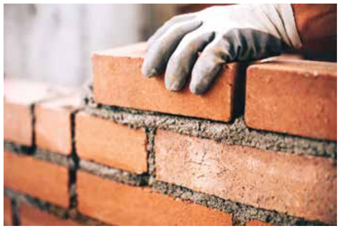
In conjunction with the appropriate protection, typical dosages of CHRYSO® Stab will produce brick laying mortars with pot lives of eight to 36 hours.
