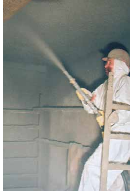
Sewament 10 being applied via spray application.
