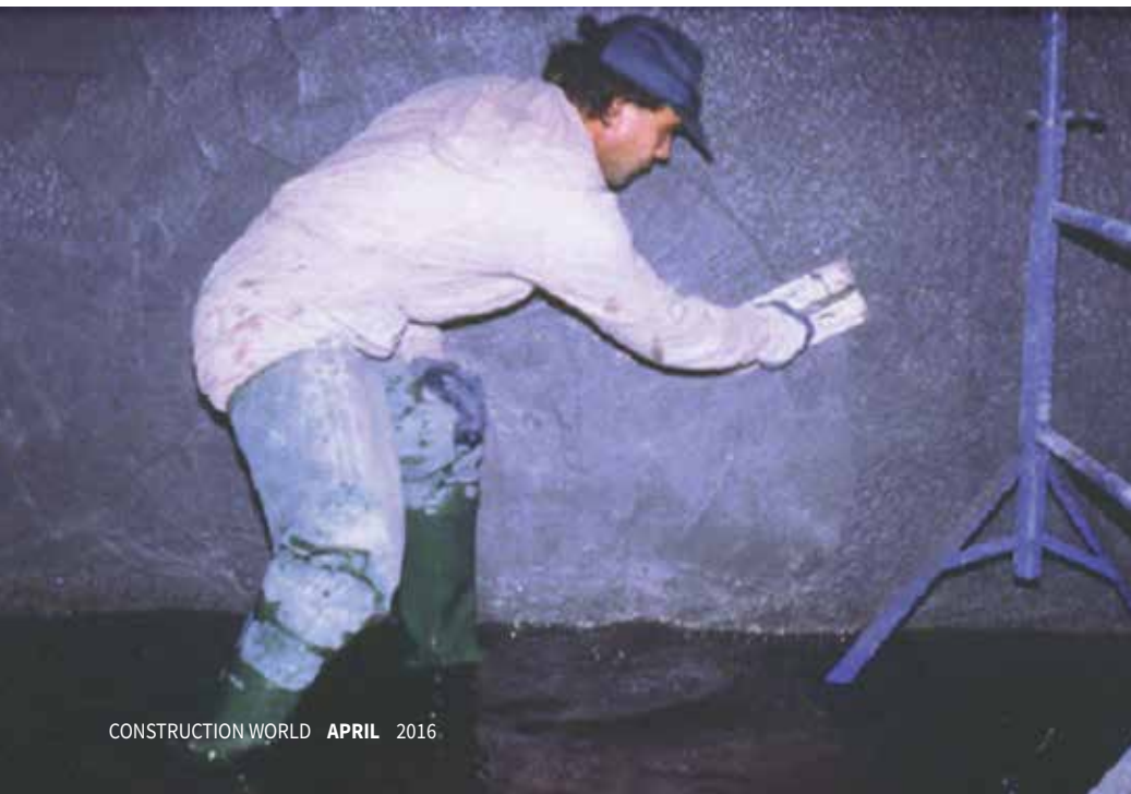
Preparing the wall for Sewament 10 application.
