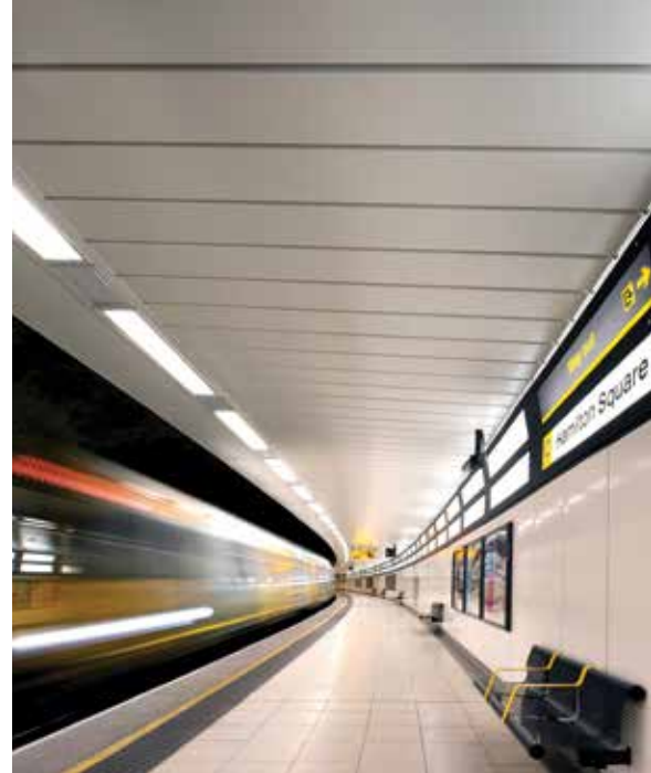
Historic Hamilton Square Station has become the fourth Liverpool tube station to be clad with vitreous enamel steel cladding supplied by the South African company, Vitrex.
