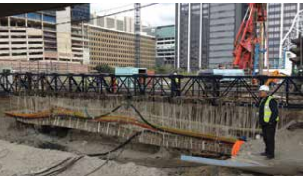
Boxed services suspended between the gravity walls awaiting slab construction.
