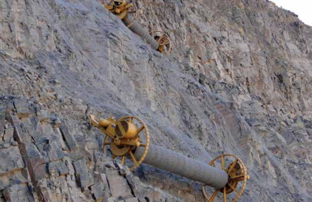
The Decoiler, 'walking' down the highwall's slope, decoiling the rolls of drape wire mesh. BELOW: The 'Decoiler', as the machine has been named, is able to handle drape mesh rolls up to 200 m in length, and 8 m wide.
