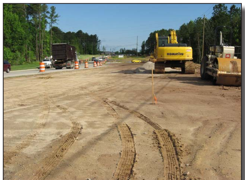
Widening of Davis Drive to four lanes in spring 2008.
