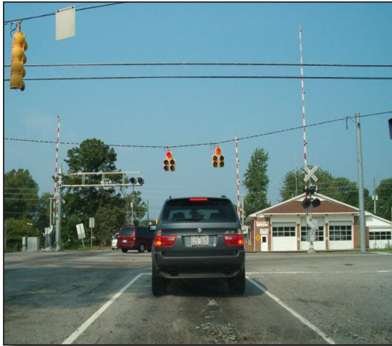
Approaching NC 54 from westbound Aviation Parkway, showing the at-grade railroad crossing just west of the intersection. This intersection is currently being improved to facilitate traffic flow.
