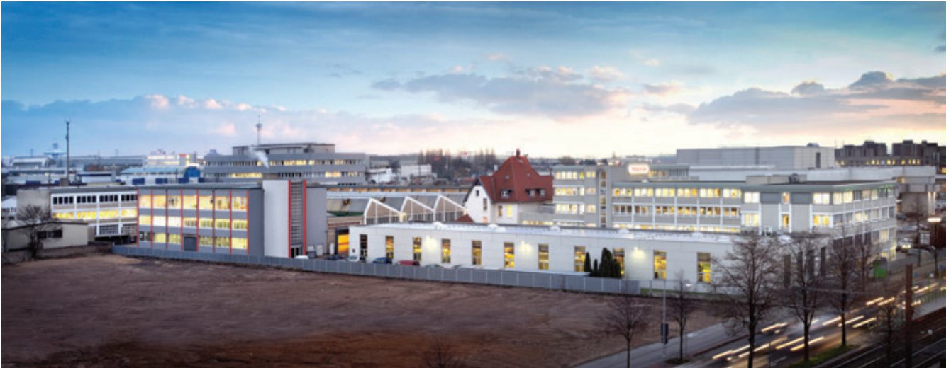
○ Troester's headquarters have been in Hanover-Wülfel since 1892
