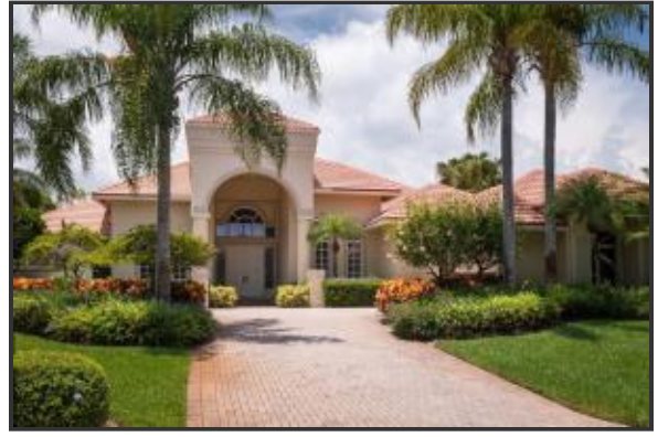
A paver brick driveway leads to the 2.5 car garage and the gracious entry doors.
