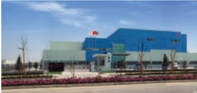
○ The new Teknor Apex plant in Suzhou, China
