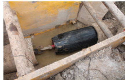
Trenchless refurbishment of old metal pipeline by 'sliplining' with PE100
