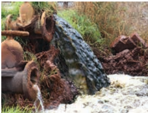
Right: West Rand, 2002 to 2016: Current AMD treatment by means of neutralisation or pH adjustment precipitates metals out of solution, which are being deposited as metal sludge into unlined pits.
