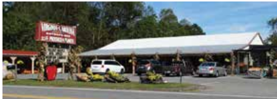
62272 - PRODUCE MARKET & GREENHOUSE BUSINESS! 20 ACRES, 3200 SQ. FT., STEEL BUILDING. $1,500,000
