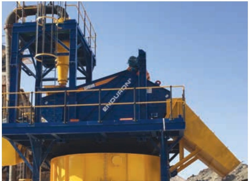
An Enduron screen being installed in a quarrying application.
