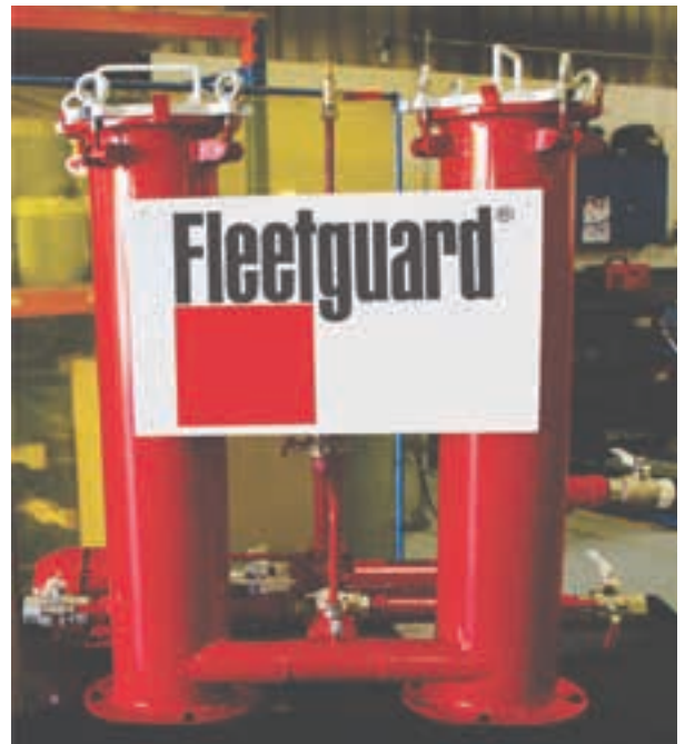
Cummins Filtration has designed and installed a bulk fuel filtration system using its Fleetguard product range to take diesel fuel from the ISO 18/16/13 cleanliness level to the ISO 12/9/6 level required at the injectors of modern diesel engines.
