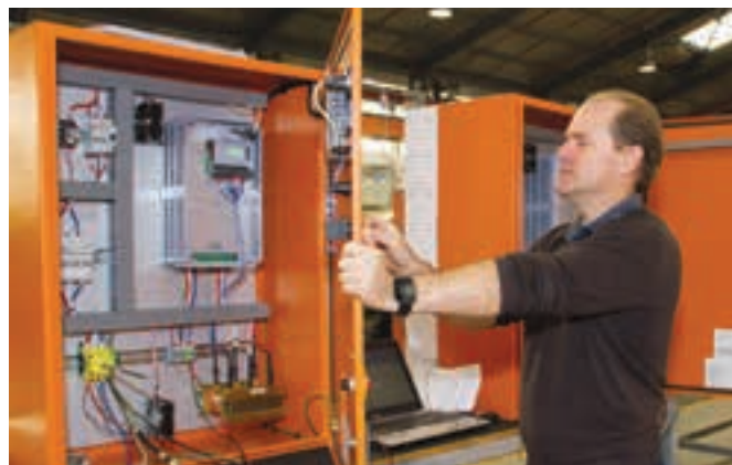
Zest WEG Group's panel manufacturing facility in Cape Town.
