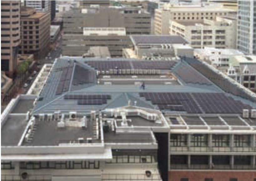
AECOM is actively working with Growthpoint Properties on a range of solar rooftop projects and existing building performance ratings, where low-performance buildings are identified and corrective measures proposed. Depicted here is the 103 kWp solar PV project at 33 Bree Street in Johannesburg.
