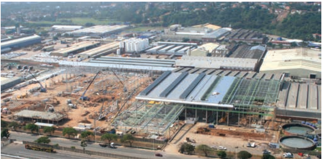
AECOM undertook the engineering services for a recent expansion project by Toyota South Africa at its manufacturing facility near Durban, including the increased capacity press shop.
