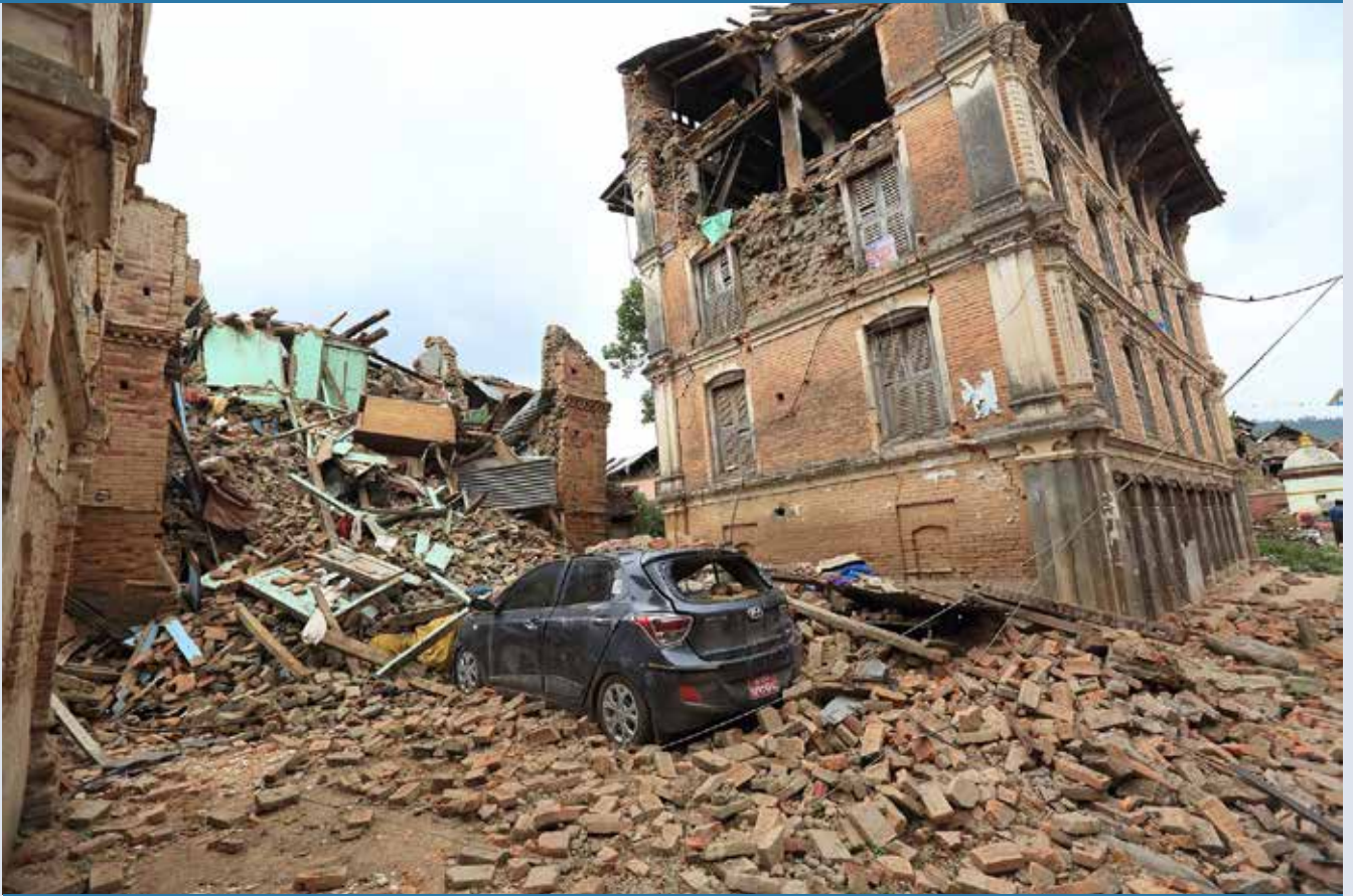
Earthquake damage in Sankhu, a particularly badly affected town in northwestern Nepal. Photo © UNDP Nepal/Laxmi Prasad Ngakhushi
