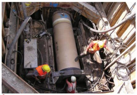
Pipes being installed in 6m depth nearby the Vistula river
