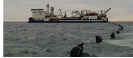
▲ Prysmian cable laying vessel Giulio Verne
