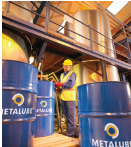
▲ One of the new blending tanks at the site
