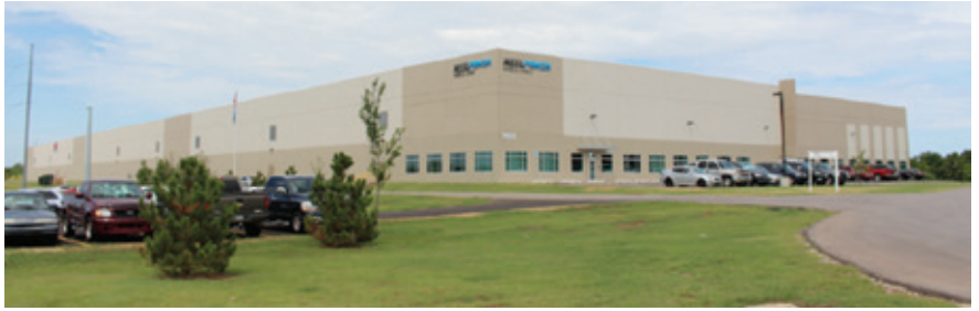
▲ The Reel Power Wire & Cable facility in Oklahoma City is the new home for Tulsa Power and Reel-O-Matic
