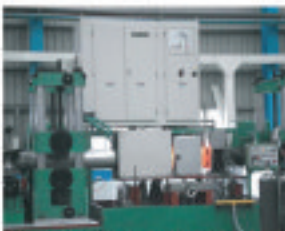
24" Pipe Mill And Annealing
