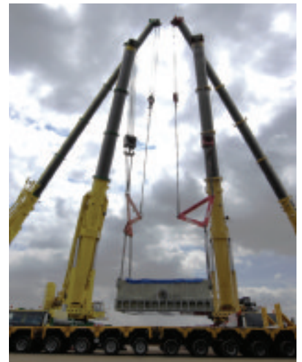
ⓘ Four heavy-duty cranes were needed to load the crossbeam onto the cargo ship
