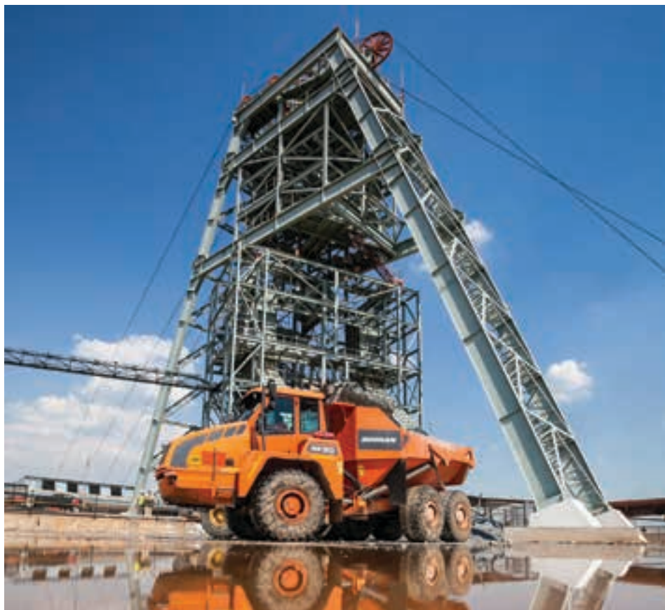
The headgear of Shaft 1 at the Platreef site (photo: Ivanhoe).
