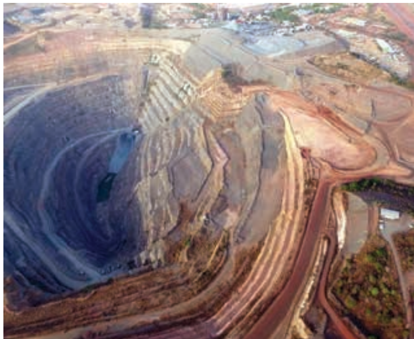
Syama open pit with main decline boxcut being developed on right of picture (photo: Rolute Mining).
