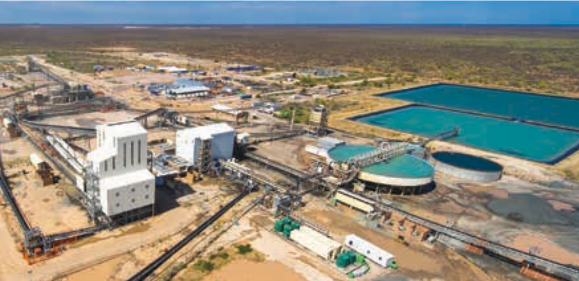
A view of Lucara's Karowe mine in the Orapa Kimberlite Field of Botswana. The tall building in the centre of the photo houses the XRT sorters (photo: Lucara).
