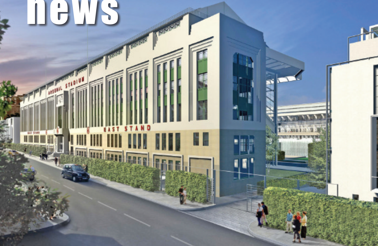
The former Highbury Stadium, transformed into 'The Stadium' residential development
