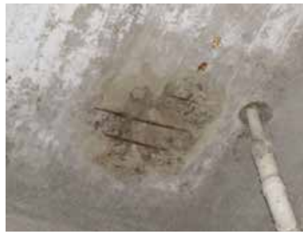
(right) Underside of a podium deck at the location of a failed expansion joint which has allowed moisture infiltration and deterioration of the supporting steel structure.
