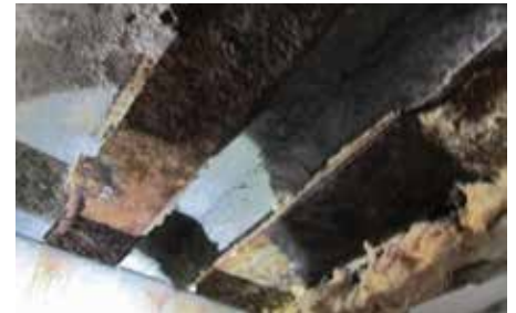
(right) Underside of a podium deck at the location of a failed expansion joint which has allowed moisture infiltration and deterioration of the supporting steel structure.
