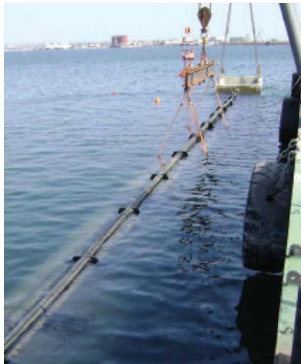
▲ Weholite, KWH Pipe's patented profile wall piping system, is easy to install on the sea floor even when the diameter exceeds two metres
