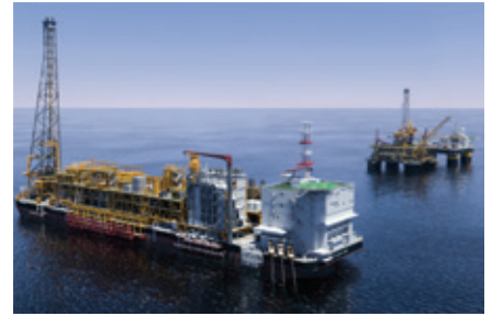
The Moho Nord project is expected to begin oil production this year
