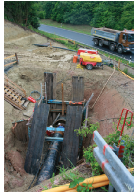
The target pit, close to a highway ramp
