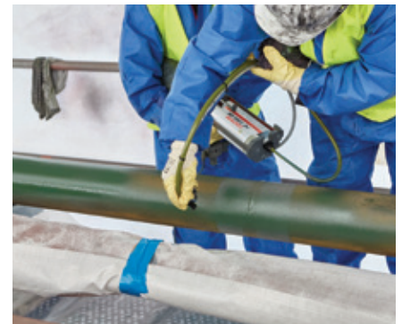
The final step in the Loctite repair system is the application of Loctite PC 7255 as corrosion protection
