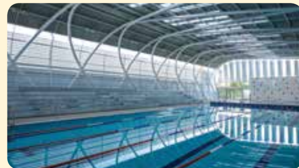
BEKA Schröder provided the lighting solution for this award-winning aquatic centre at the American International School of Johannesburg.
