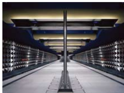
Stainless steel wall cladding, Poliant-coated to improve cleaning properties
