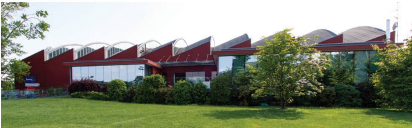
▲ The new headquarters in Castellanza, Varese, Italy
