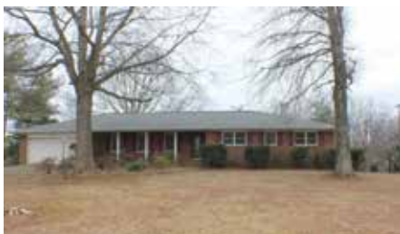
875464 - 150 DEVOTION - Beautiful brick ranch home on 1.63 acres with extra storage/workshop building with shed. The home has 3 spacious bedrooms, large living room, beautiful oak cabinets, large laundry room, attached garage, partially finished basement with half bath and bonus room. Must see to appreciate this beauty as it sits in a very scenic country setting with distant MTN views. $147,500
