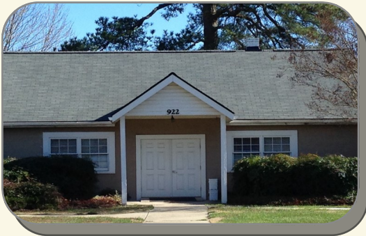
Luther Green Center Roof Replacement
