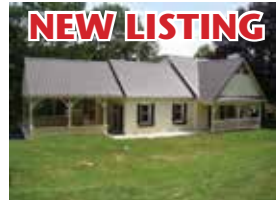
2131 - HILLSVILLE - REMODELED HOME, TOWN LIMITS, 1546 SF, 3BR, 2BA, NEW FLOORING ROOF AND DECK, UPGRADED ELECTRICAL AND PLUMBING. $144,000
